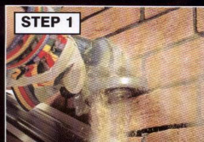
Chase out with grinding wheel
