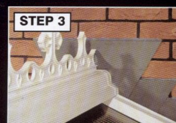
Install pre-formed apron flashing and silicone the joint
